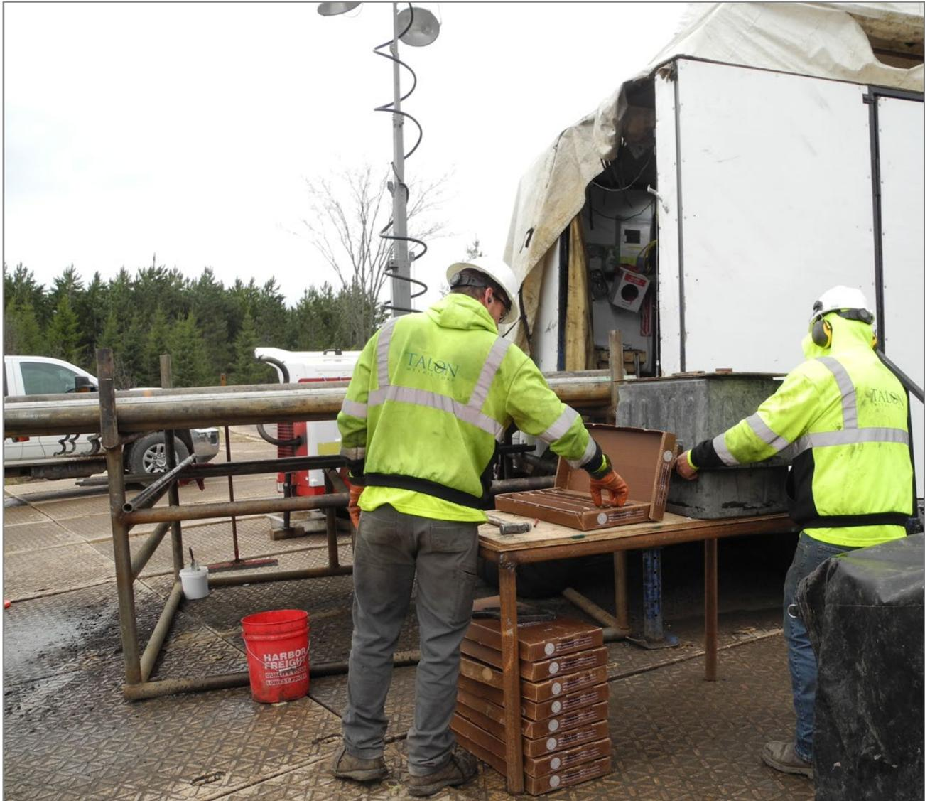
**Figure 12.8: Digital Photography of Core in Box Beneath the Black Bin Apparatus, with Drill Crew Sending Photograph via Commercial Cellular Network to a Talon Server.**
