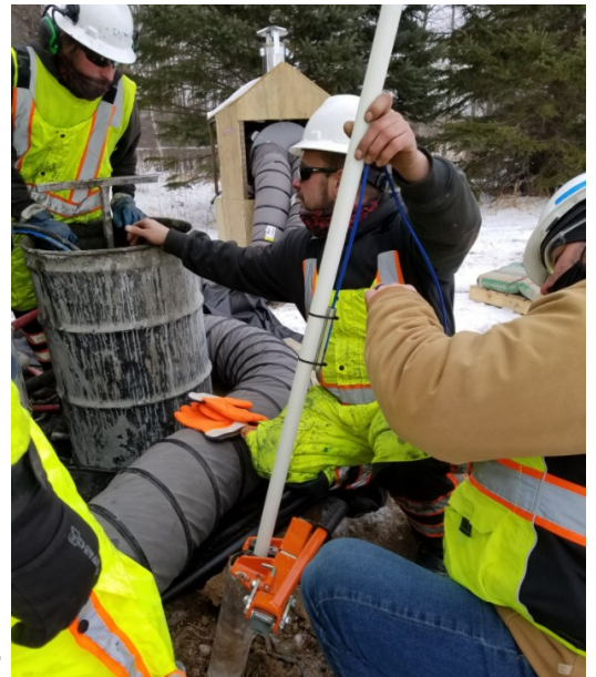
The Talon team installing the piezometers.
