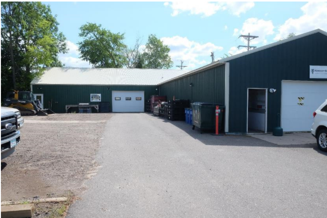
Figure 11-1: Photo of Kennecott/Talon Core Processing Facility Tamarack, Minnesota
